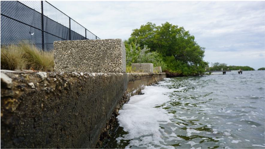
The existing concrete seawall on the north end of Bayfront Park will be replaced with a sloped living shoreline. Photo by Carter Weinhofer
